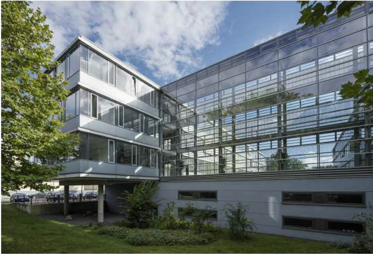
The Potsdam Centre for Technology, the registered office of Runge
